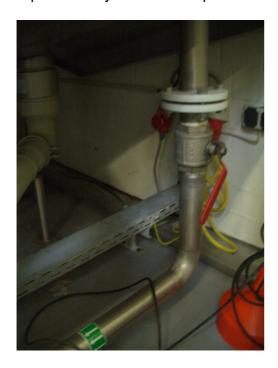
Inflow of pre-cleaned water out of recycle flow towards the pump
